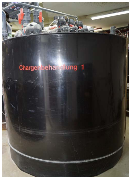
Photograph shows wastewater holding tank.
